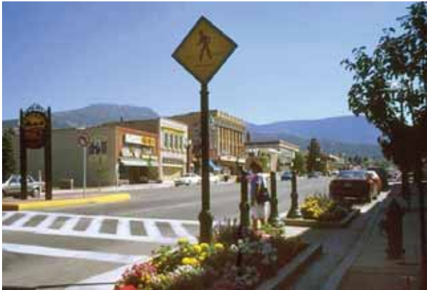
This wide Main Street in a historic town has been improved with the addition of medians and parking-lane landscaping at a midblock crossing. The curbed planters have been cut through at the crossing and along the curb to maintain drainage; the edges provide good non-visual wayfinding cues. Still needed: detectable warnings at the street edge, where there is no indication of the change from pedestrian to vehicular way.
