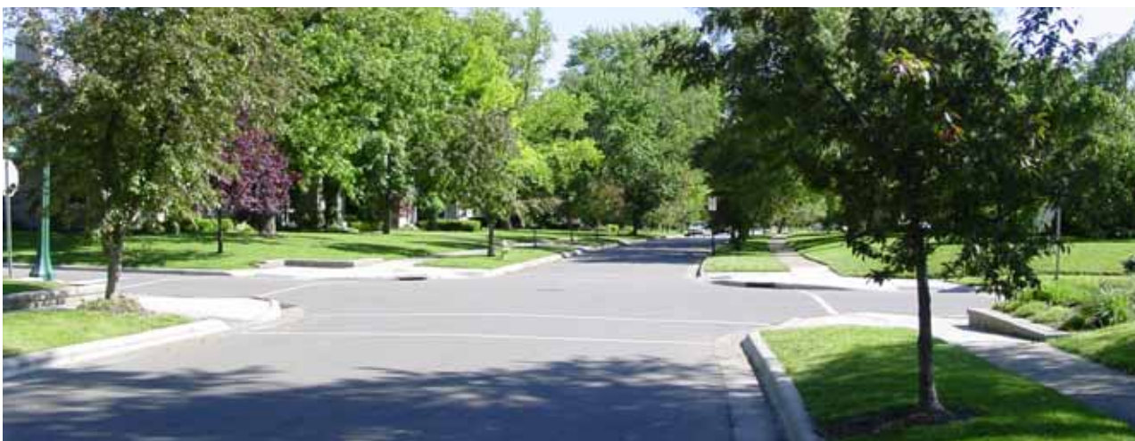
This reconstructed residential street in Ohio curves through several intersections skewed by as much as 30 degrees. Although aesthetically pleasing, this posed some design challenges for accessibility. As can be seen in the photograph, low retaining walls were required on many corners. The project included new water mains, fire hydrants and services, sanitary and storm sewer rehabilitation, new curbs and gutters, driveway entrance replacements (to allow ADA-compliant sidewalks across the driveways), and full-depth street reconstruction for approximately 1.5 miles of suburban streets. Paired curb ramps with detectable warnings were constructed at all intersections.
