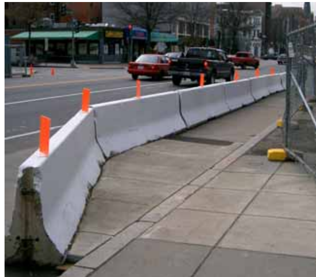
This urban arterial passes through a neighborhood that is undergoing rapid revitalization, with many projects under construction temporarily occupying existing sidewalk space. In this example, the contractor has provided a temporary pedestrian route in the curb lane of the roadway, separating it with Jersey barriers and installing a temporary concrete ramp to the street level walkway. Still needed: detectable warnings at the cross street.
