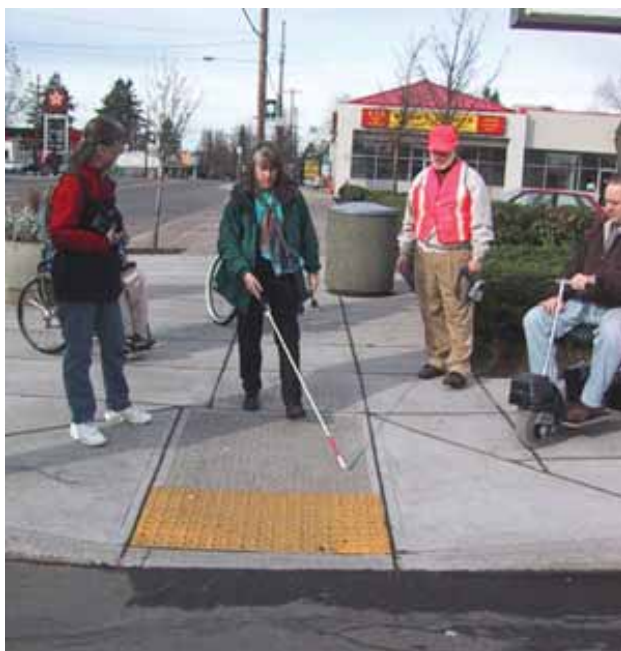
PROWAAC members observe a thin-film detectable warning retrofit on an existing curb ramp in a pilot project in Portland, OR
