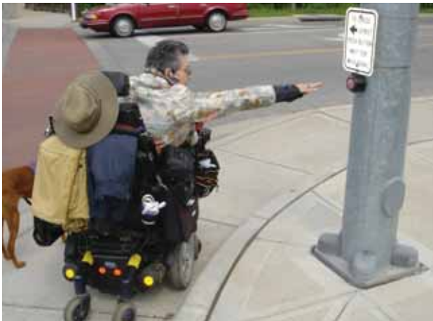
This new parallel curb ramp on a large-radius suburban corner curves down to the street and is otherwise usable, but the pedbutton isn't. Installed on a signal pole, it is out of horizontal reach range for this pedestrian. A better installation can be seen across the street, where a stub pole has been installed in a more usable location.
