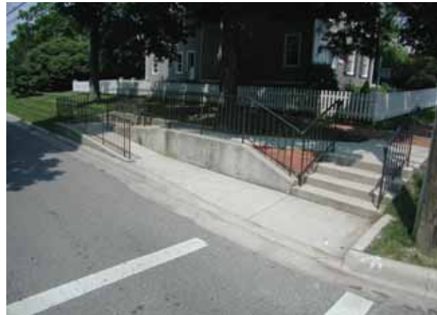
Sometimes difficult topography requires extraordinary solutions. In this photograph of an older Ohio residential neighborhood, the existing roadways are much lower than the sidewalks and separated by wide sloping lawns. New stairs and ramps—both with handrails—make the connection to the street crossing for pedestrians.
